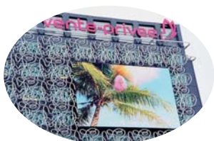
headquarters "Vente-Privée" (Paris 2015) concrete molding, RAIGI formulation
